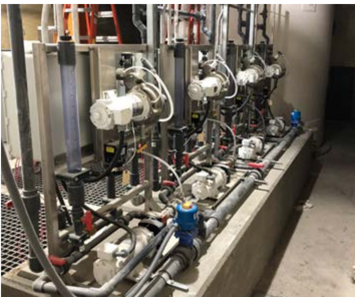
Wichita WWTP#2 – Polymer Feed Pumps
